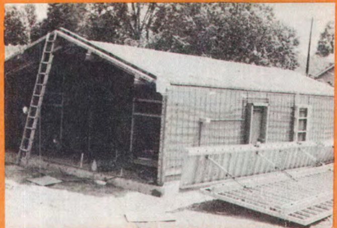
The inner forms, wheeled onto the floor slab and positioned by a simplified system of screw-jacks, hold roof forms in place and will be removed after house is poured.
