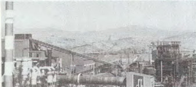
Copperhill operations' new smelting operations are shown in this picture. At left is the iron pelletizing plant, the iron and copper facilities are located in the center portion and the huge duct leading off to the right carries the sulfur dioxide gases from ore smelting operations to the acid plants.
