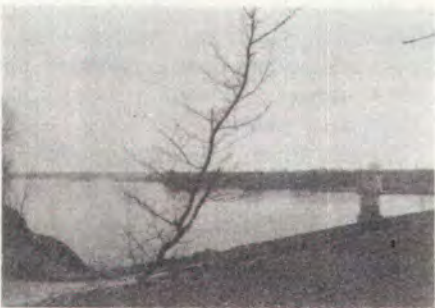
Views at dam looking toward the reservoir area on December 2, 1970, only one day after the valves were closed to start the filling of the lake; January 15, 1971; February 14, 1971; and March 12, 1971.
