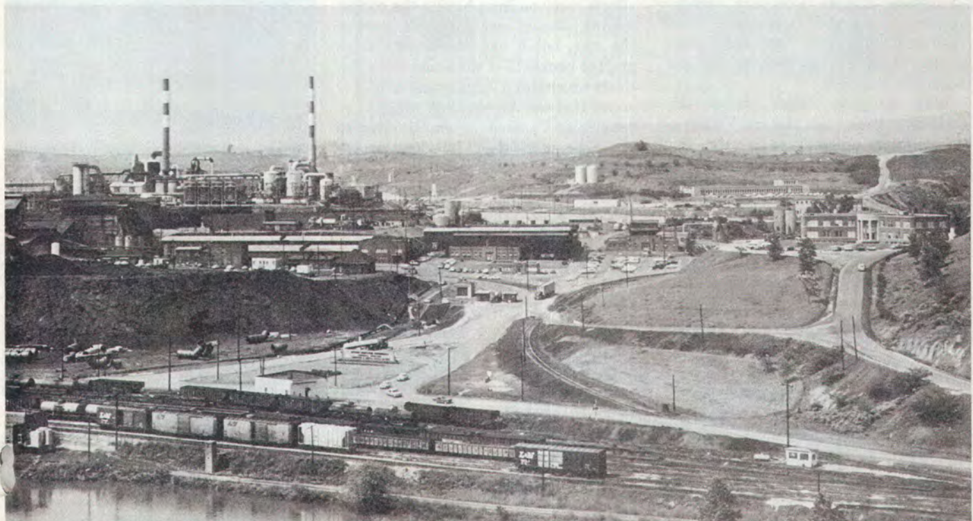
General view of Copperhill plant looking through main entrance. At top left are some of the acid producing facilities and the general office is at the extreme right in photo.
