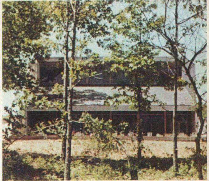
The new commons building, viewed from nearby Barkley Lake, serves as headquarters for the Brandon Spring Group Camp.
